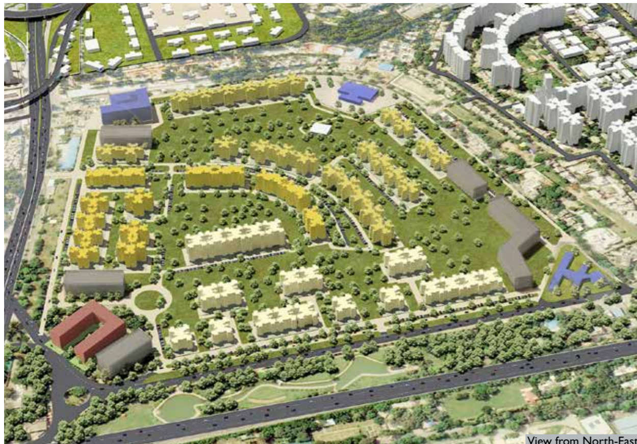
View from North-East
